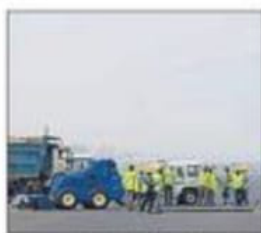
The runways 09/27 and 14/32 will undergo repair work.
